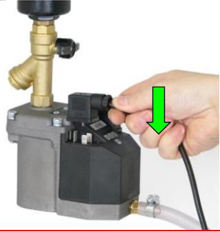
25. Restore POWER supply. Check if the power LED lights up to confirm correct electrical installation.
