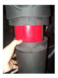
Open the thermal insulation at the filter head and remove the portion of the insulation relative to the filter body.
