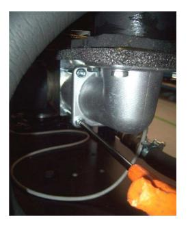
Remove the no-return valve from the aluminum casing and replace it. Pay attention to the direction of installation of the no-return valve; the rubber coated part must be positioned on the elbow side (see picture).
