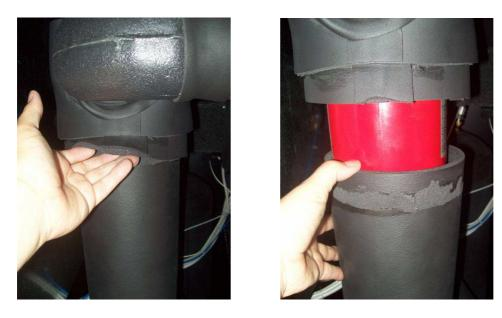
Open the thermal insulation at the filter head and remove the portion of the insulation relative to the filter body.
