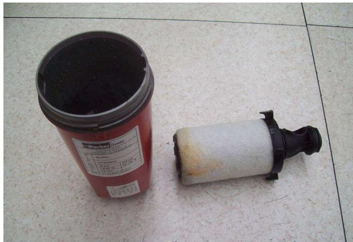
Slip filter body from the head, extract the filter element and replace it.
