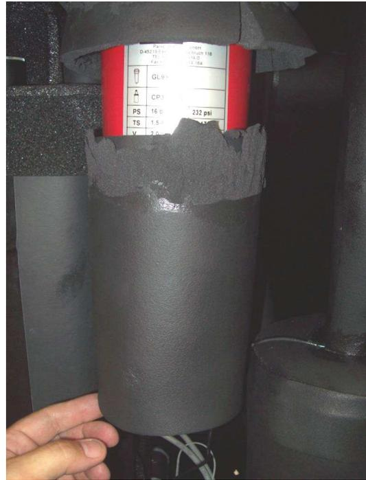
Open the thermal insulation at the filter head and remove the portion of the insulation relative to the filter body
