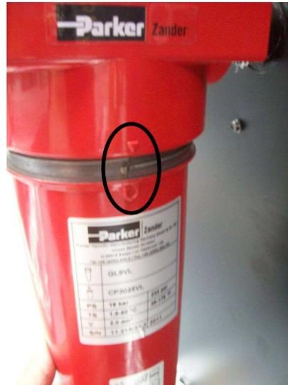
From the initial position (reference marks aligned), turn the filter body one full turn to re-align the ref. marks.
