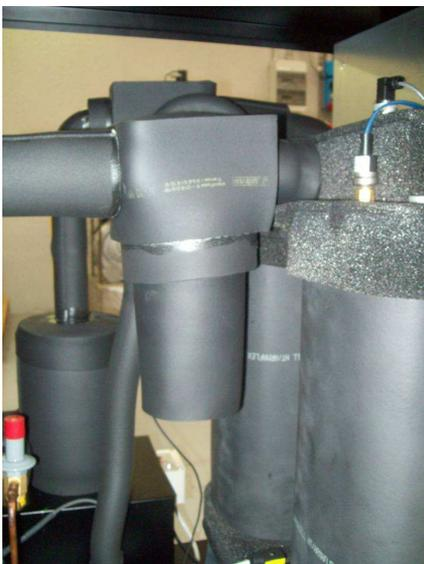
Reapply the thermal insulation previously removed (paste it if necessary).
